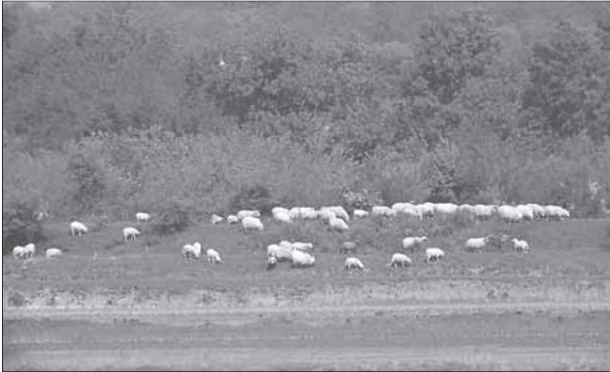
Fig. 16: The Solana's outer dam is grazed by free-roaming sheep. 25 April 2003, Solana Ulcinj (Photo: P. Sackl).
