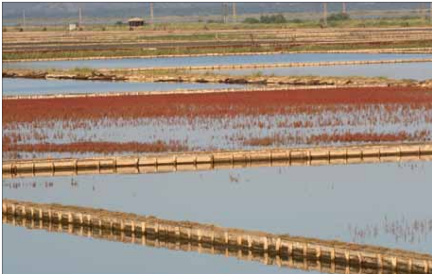
Plate 2: Small, almost rectangular crystallisation basins characterize the pans of the highest evaporation grade. 19 June 2008, Solana Ulcinj (Photo: T. Petras-Sackl).
