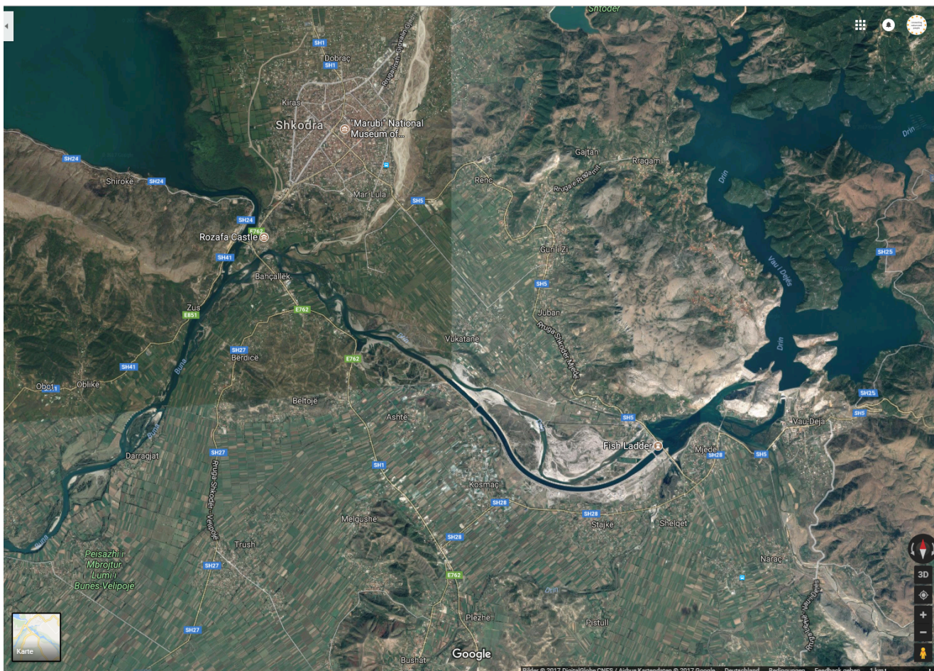
Figure 1: The project site at the Drin river close to Lake Skadar with the bypass canal.
