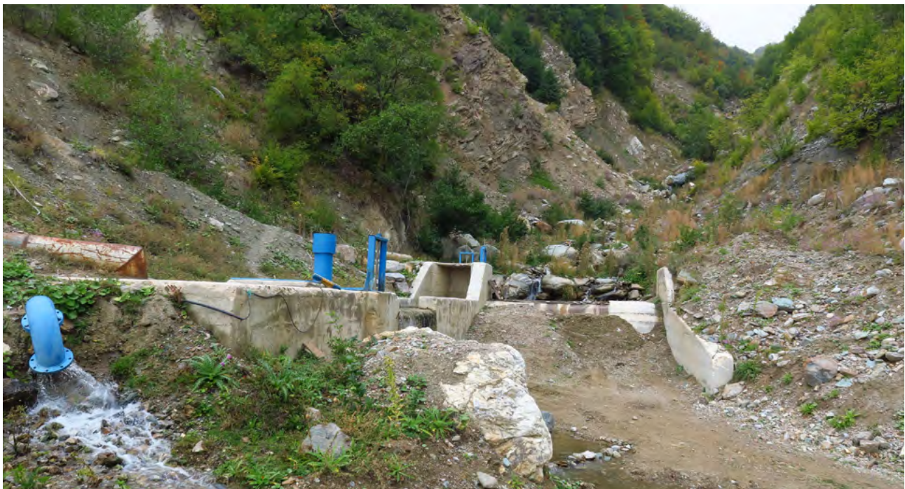
Brza Voda 2 intake with no fish pass, North Macedonia
