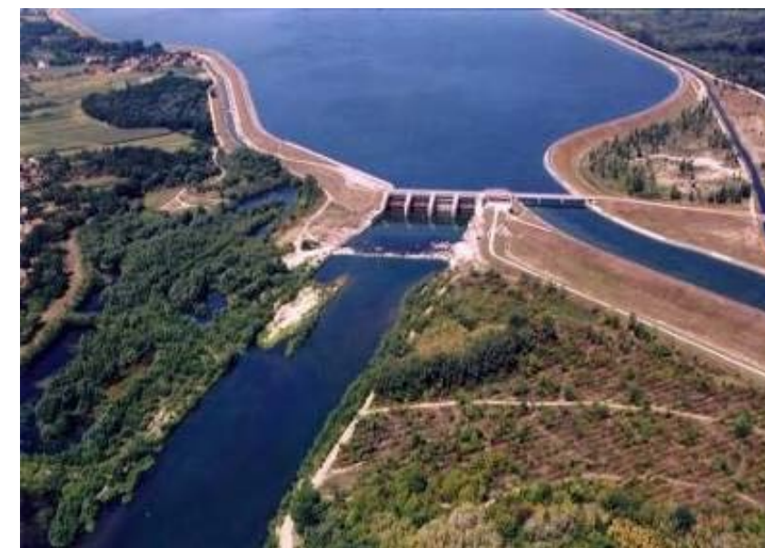
Fig. 27: Typical situation of a diversion dam system on the Drava at Varaždin: The Dam reservoir covering the whole former riverine landscape; bypass canal to the power house (energy production) on the right side and release channel for flood situations on left side (Credit: WWF)
