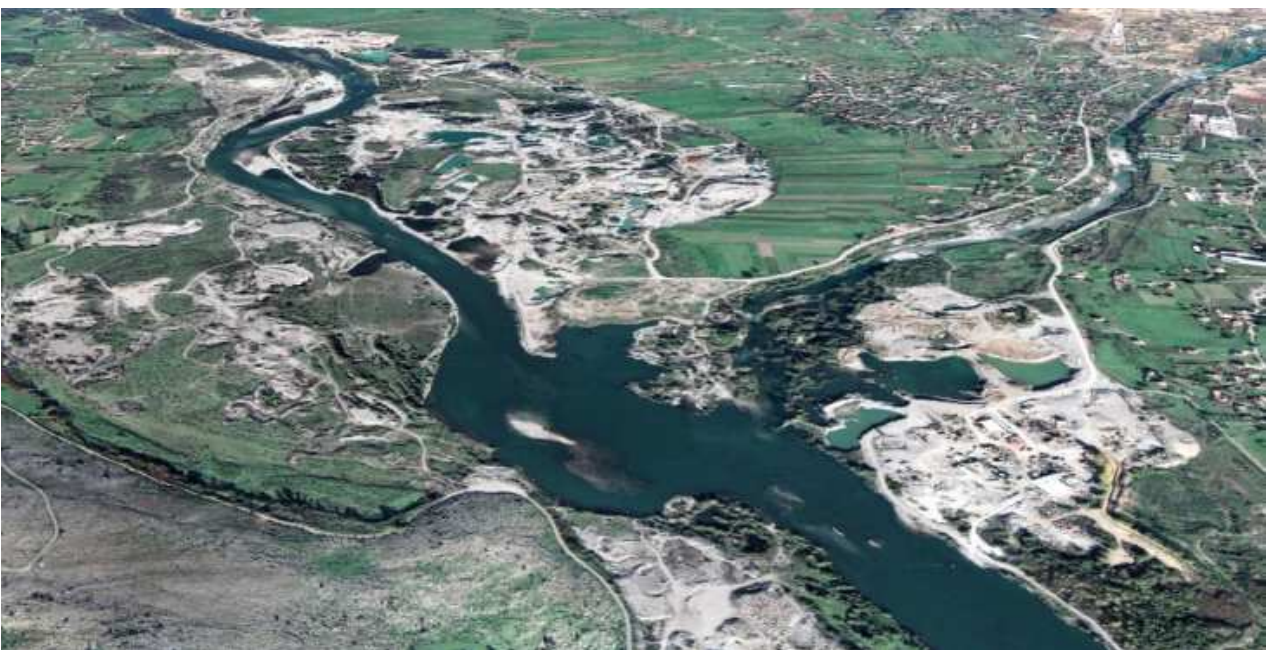
Figure 7: Excessive dredging in lower courses contributes to sediment transport deficits causing incision and degradation of deltas (example from Morača River, Montenegro) (Google Earth 2023).
